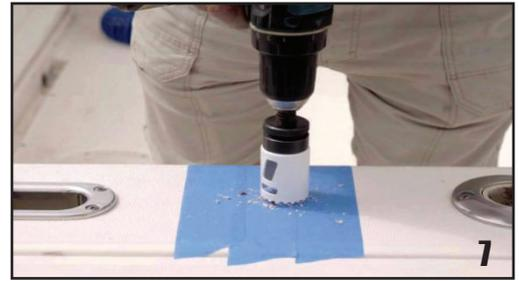
7) Cover area selected to mount the Receiver with marine masking tape. Using the drill and 1 ½" hole saw, cut hole in designated area to mount the Receiver.
