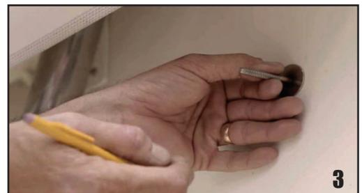
6) Apply JB Kwikweld to stud base and place the stud on the area previously prepared. Push the stud firmly in the desired location and turn it ¼ of a turn. A piece of tape can be used to hold the stud in place until the JB Kwikweld sets up.
